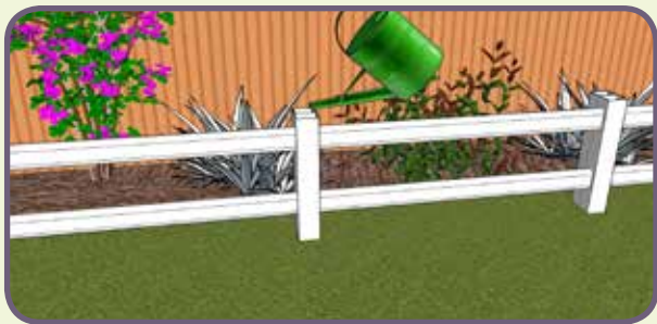
7. Fill to the top of post with water to set the sand.
