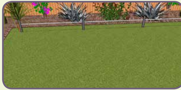
2. Hammer in angle irons until half way into the ground.
